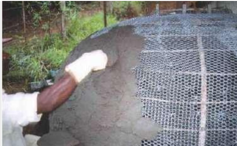
Fig-14 ferro concrete
