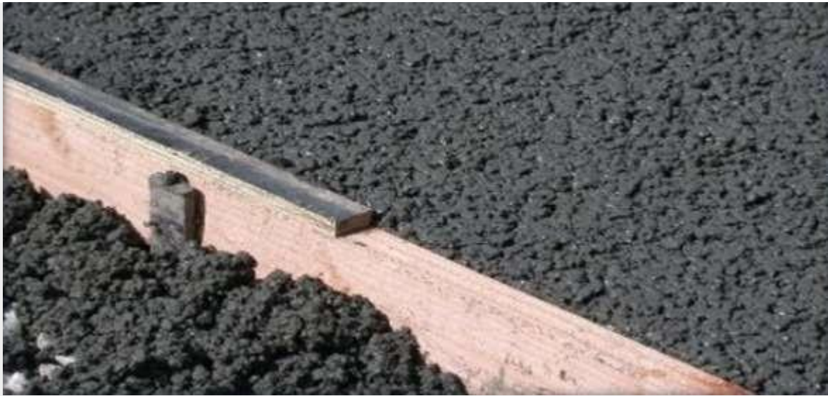
Fig-7 No Fines Concrete
