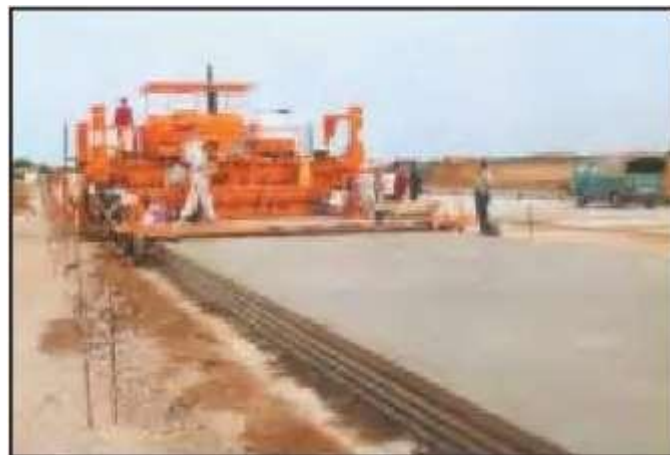
Fig-6 placing of concrete
